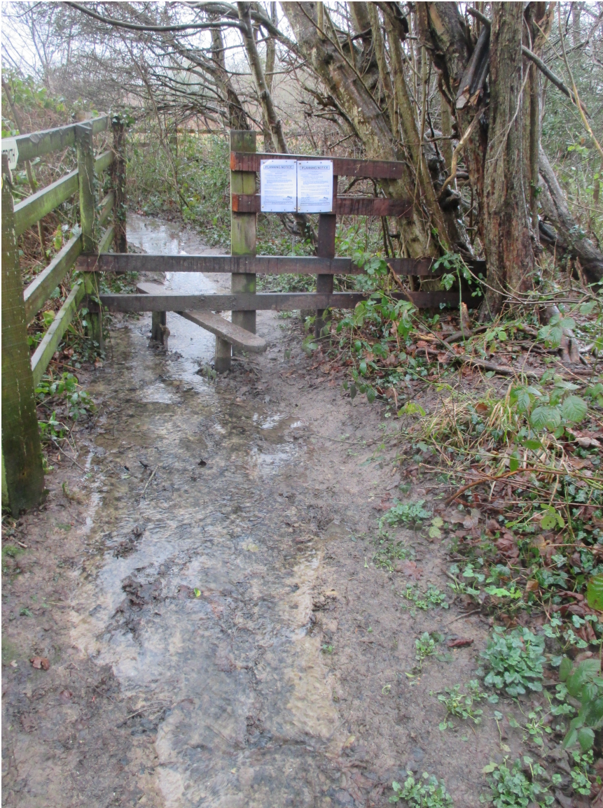
Figure 19 - Overflowing SUDs scheme in Juziers Drive flooding the Public Right of Way.
